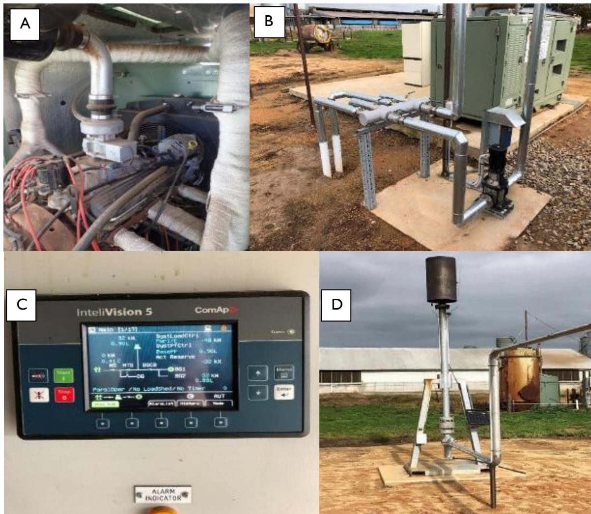
Figure 5 Photos of the biogas-fuelled combined heat and power engine generator (A, B, C) and the emergency flare (D). The respective photos show (A) the generator unit when originally purchased second-hand with wear and tear due to disuse and (B) after retrofitting and installation at the case study piggery, (C) the control system screen, and (D) the solar-spark partially shrouded emergency flare. The flare has a thermocouple to confirm whether the flare is operational by measuring the presence of a hot flame.
