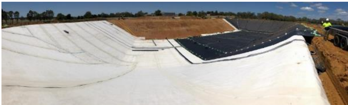
Figure 7 Example in-ground dam lining performed by Waterlogic, showing liner on the left and geotextile protective layers (Source: Waterlogic).
