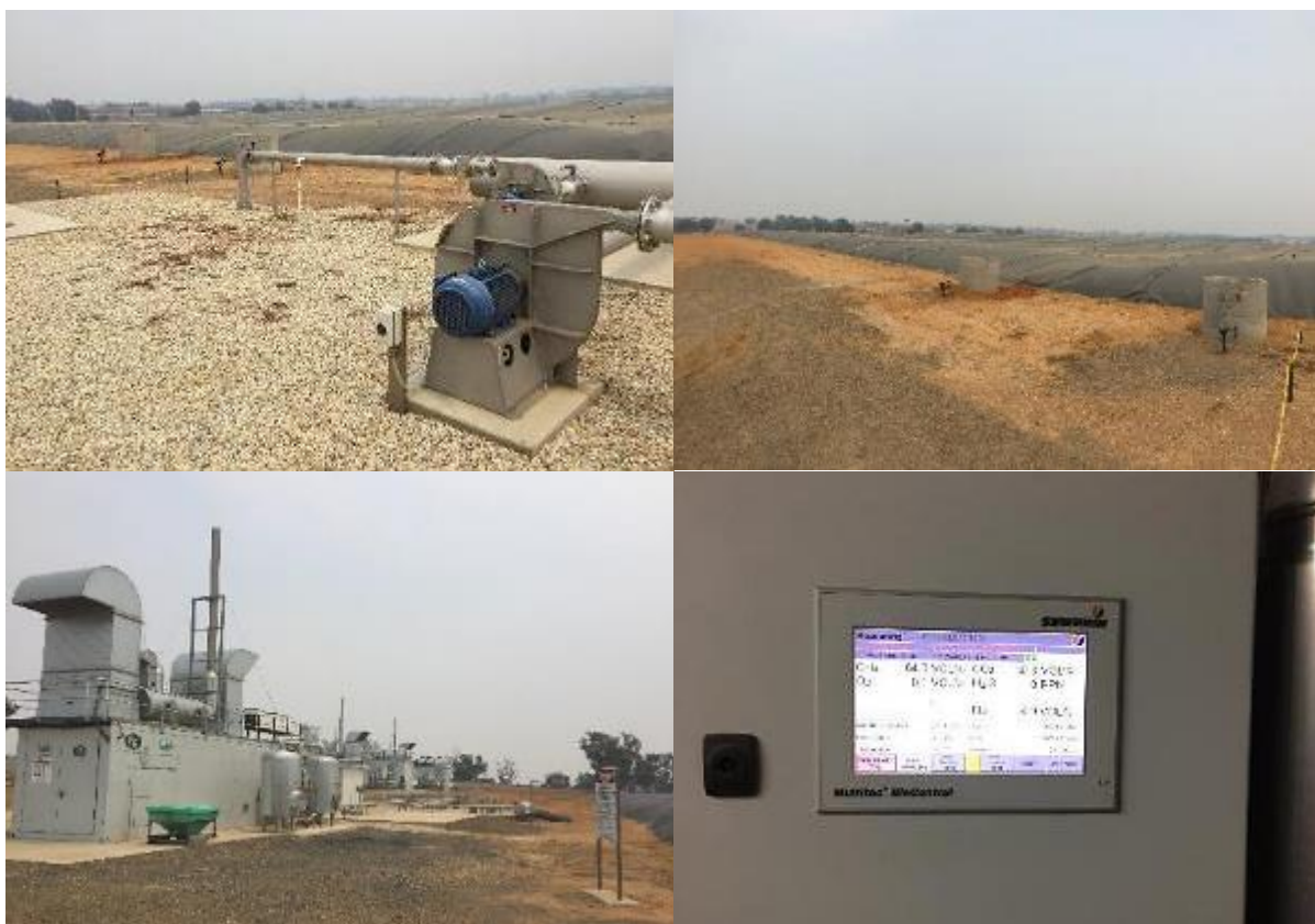
Figure 11 Photographs of biogas infrastructure, taken during the project site visit. The infrastructure includes two covered anaerobic ponds (top) and three 500 kWe Evo 2G generators (bottom left corner), producing electricity with biogas containing about 65% methane (bottom right corner).
