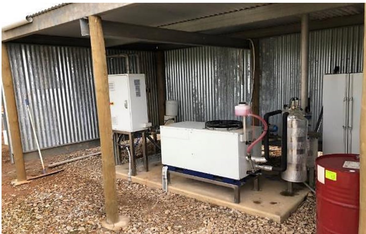
Figure 4 Electrical chiller (not absorption chiller) and shell and tube heat exchanger used to condense and remove moisture from the biogas prior to use at the case study piggery.
