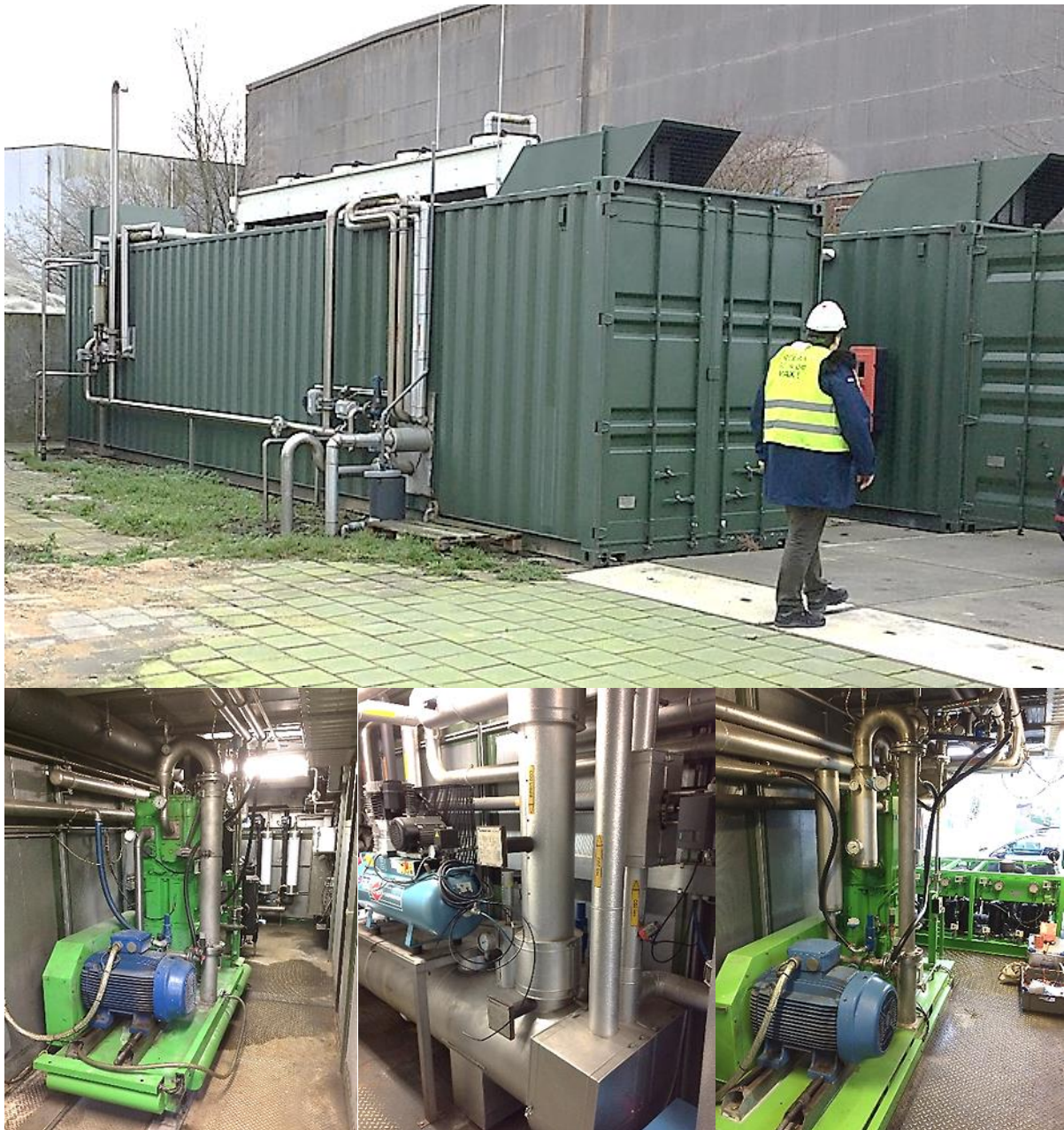
Figure 14 Example membrane-based biogas upgrading infrastructure in the Netherlands, by Pentair Haffmans. The infrastructure is fully containerised inside pre-assembled 40-foot containers, making it modular and readily transportable. Photos also show infrastructure inside the containers, including a compressor and membrane units for separation of methane from \text{CO}_2 (left), heat exchangers (middle), and refrigeration units able to produce liquid \text{CO}_2 . This example system is identical in size to what would be suitable for the large piggery concept, i.e. 250 \text{ m}^3\cdot\text{hr}^{-1} raw biogas flow. Source: Tait (2018).
