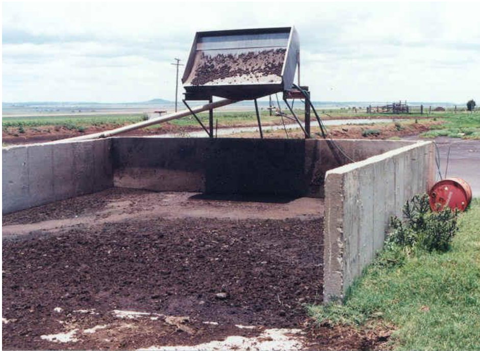
Photograph 1: Collection of thickened solids from a static screen
