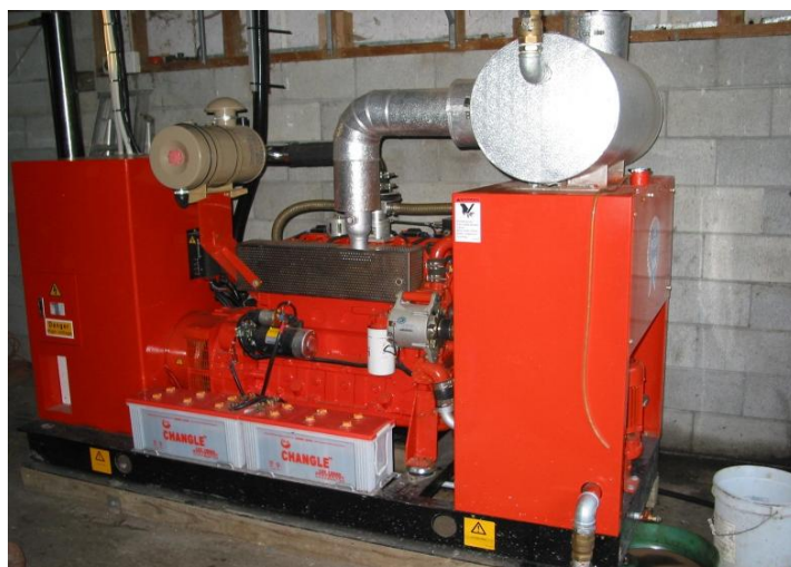
Photograph 4: 48/40 kW 6-cylinder spark ignition CHP biogas generator at the Lepper piggery in Taranaki, New Zealand.
