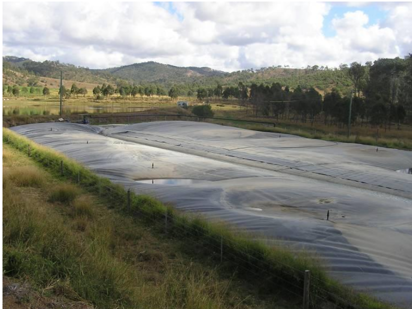
Figure 7: A covered anaerobic pond (CAP) installation at an Australian facility
