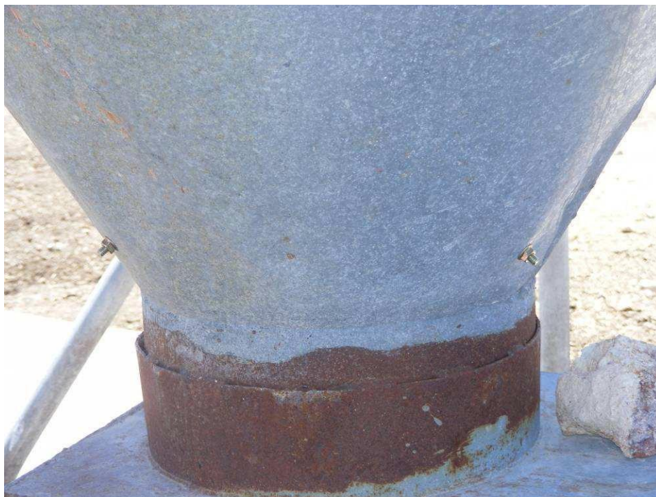
Image 4: The bolts visible on the outside of the cone indicate where the Sure-Flo® silo insert sits in the silo. The product brochure suggested that the insert should be down in the collar or neck of the silo.
