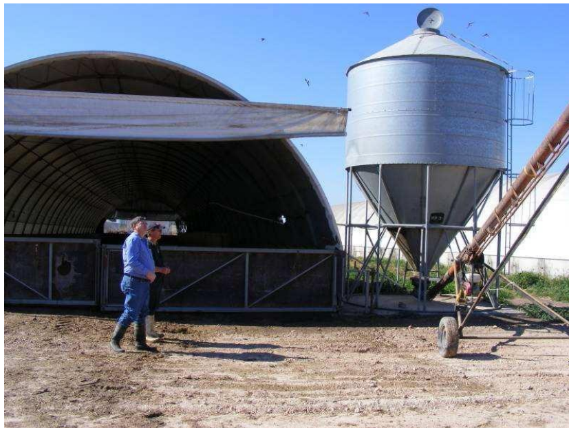
Image 6: One of the large silos relative to shed – its cone looks to have the right angle to encourage mass flow. Greg Mills and Geoff Fisher in front of shed.
