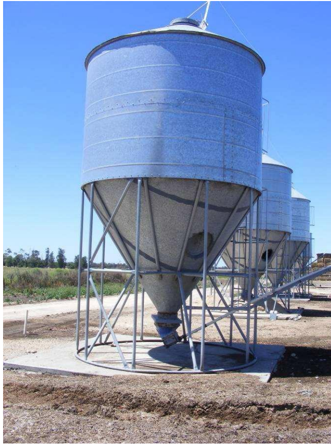
Image 5: Cone angle is important for good flow – for mass flow to occur the recommended angle is 40^\circ from vertical axis (Chase Akron University) – these silos appear to be of the right shape. This is a photo of some of the small silos.
