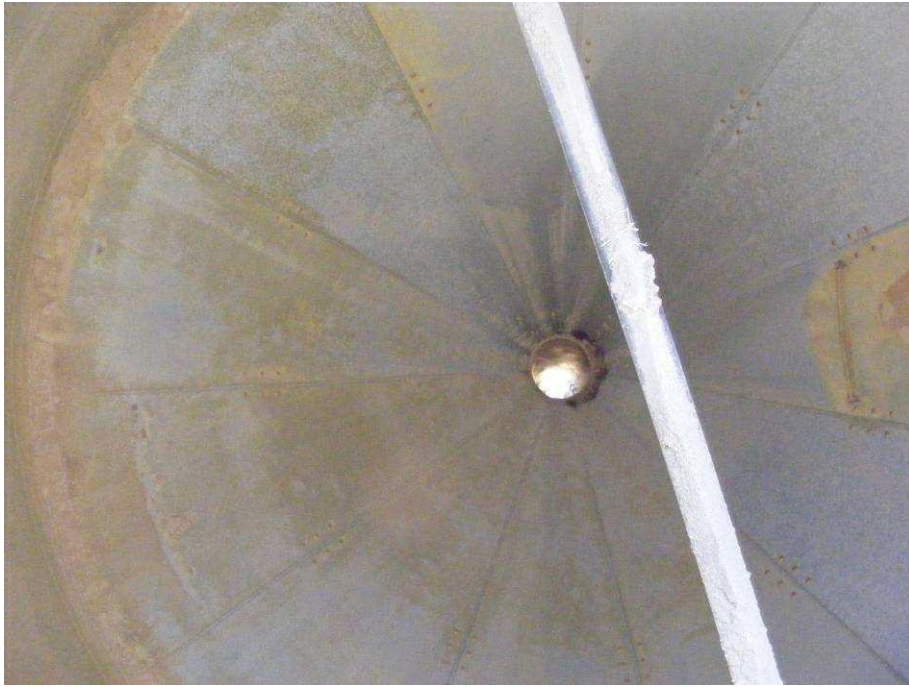
Image 7: There is less resistance to flow if the walls are smooth and shiny. The internal surface in this silo cone almost looks rusty in places.
