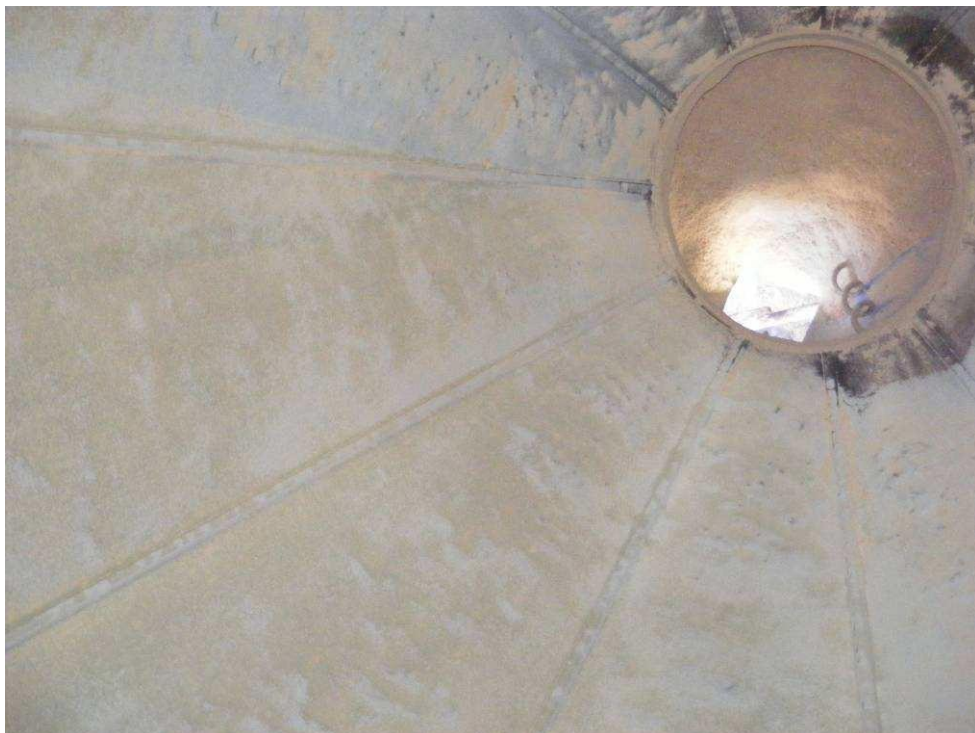
Image 8: Feed residue on walls of the cone has collected in the dents resulting from knocks to the cone walls over the years.
