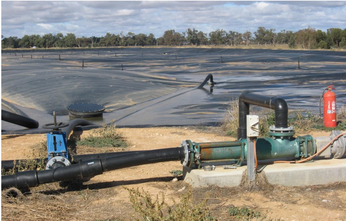
Figure 3: Original sludge extraction pump (previous location at inlet end)
