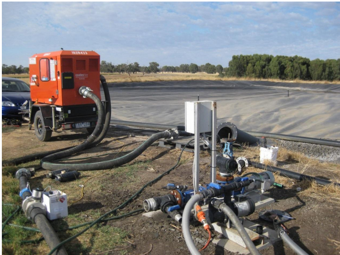
Figure 11: Hire pump operating from the inclined access sleeve, February 2013
