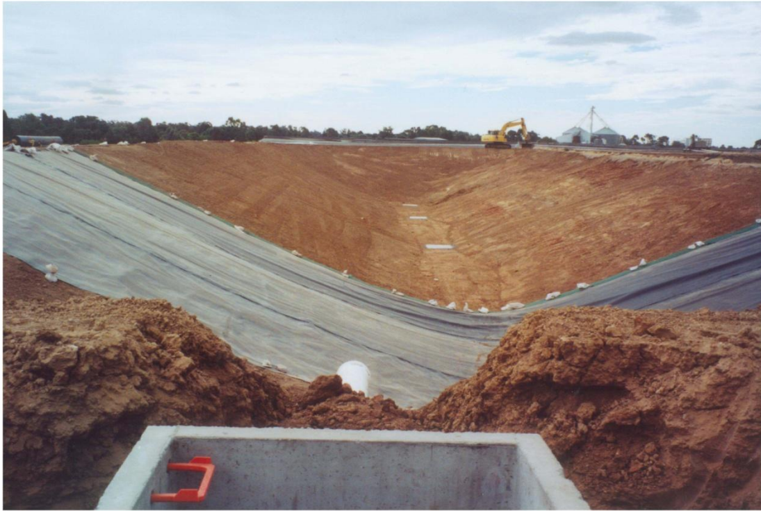
Figure 2: The completed earthworks with cover shown prior to floating (2004)
