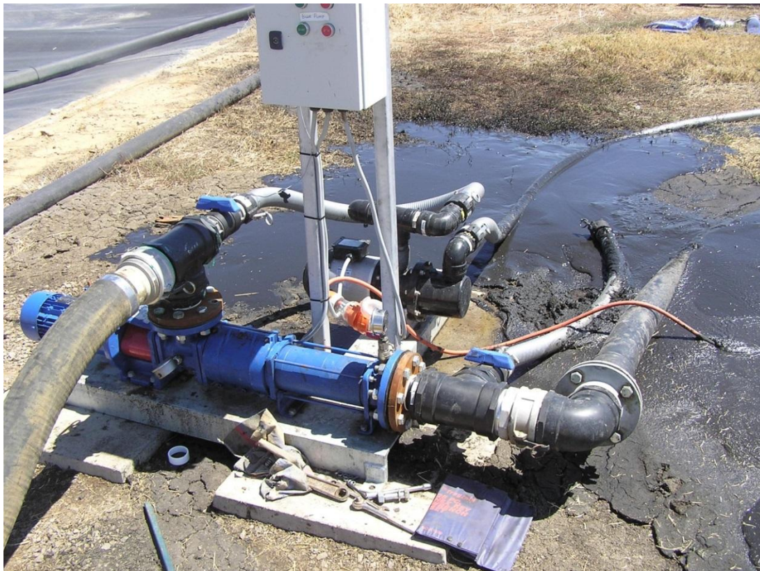
Figure 10: Replacement desludge and backflush pumps, February 2012
