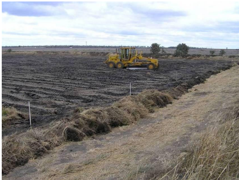
Figure 2: Stripping piggery solids from the base of the disused effluent evaporation pond in preparation for construction.
