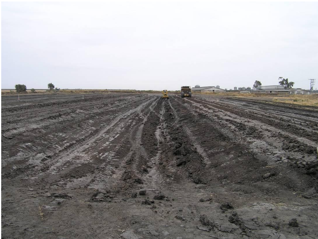
Figure 4: A grader was used to trim the earthworks following placement with the scraper and compaction using the vibrating pad-foot roller.
