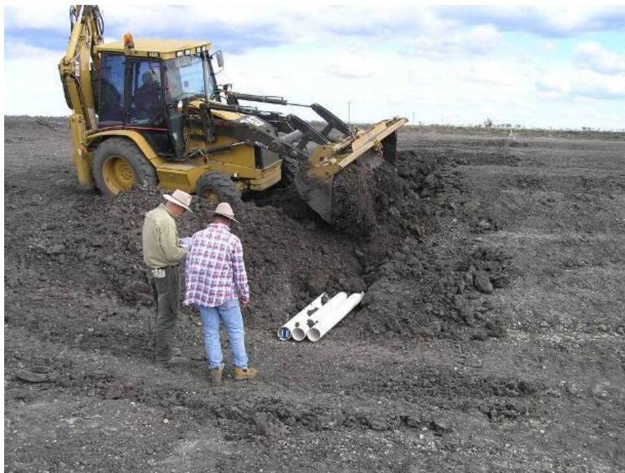
Figure 8: Backfilling the pipeline trench where the three SEPS drainage pipelines enter the return drain.
