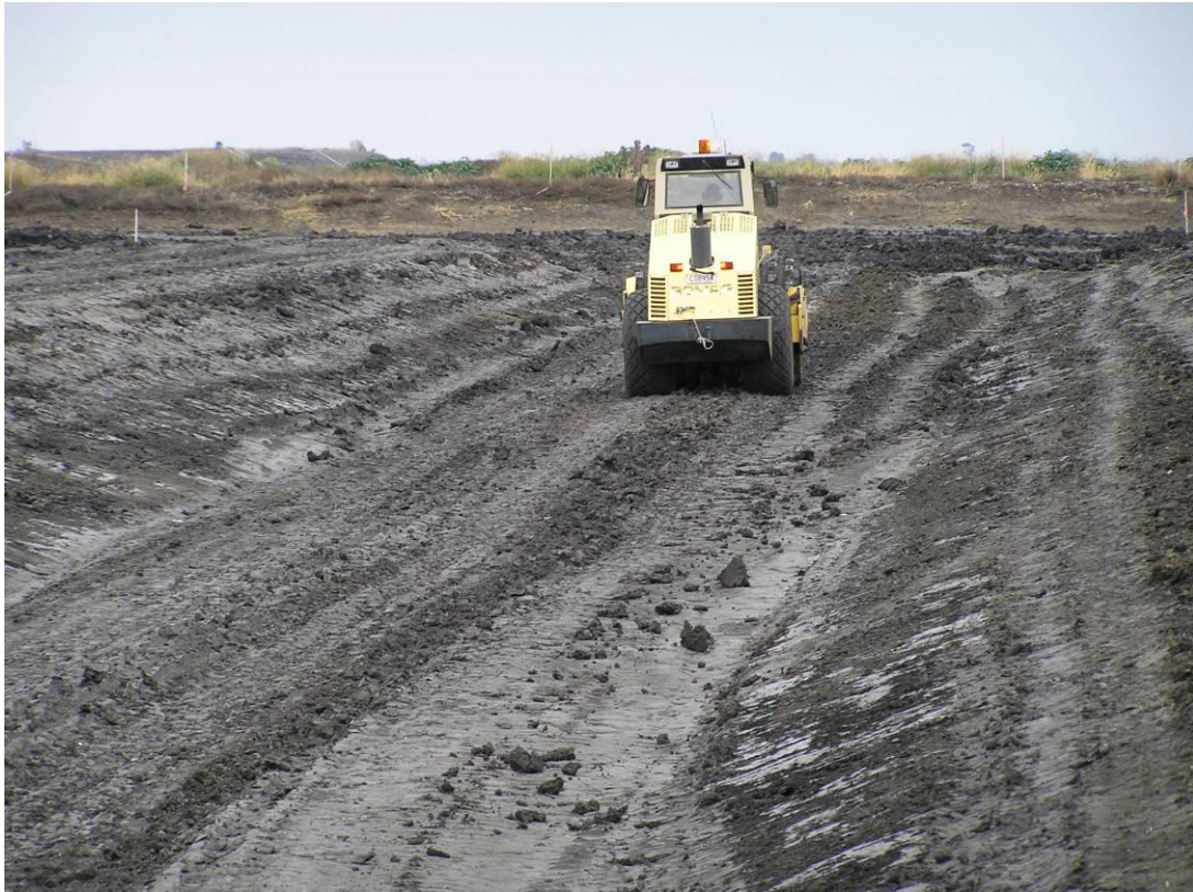
Figure 5: Vibrating pad foot roller compacting the base of one of the SEPS channels
