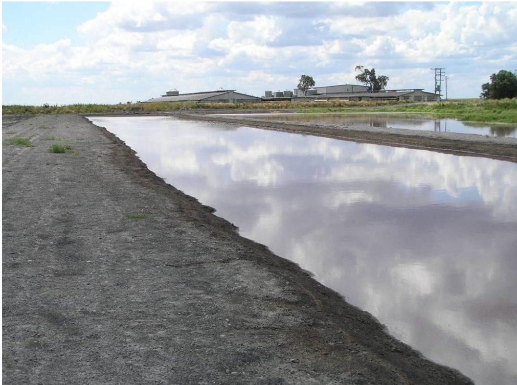
Figure 12: Photograph of the first SEPS channel and return drain on 5 November 2009, after approximately one month of active operation.
