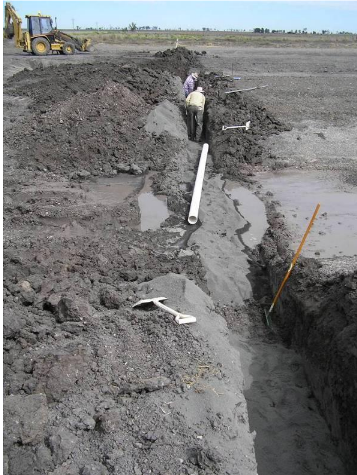
Figure 7: Laying individual 150 mm diameter PVC drainage pipelines from each of the SEPS channels to the return drain.
