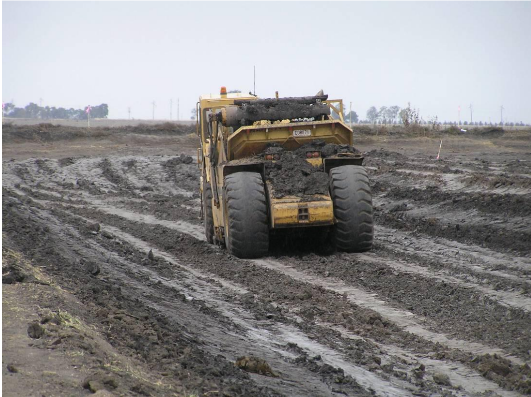
Figure 3: A scraper was used to remove material from the base of the SEPS channels for placement on the banks.
